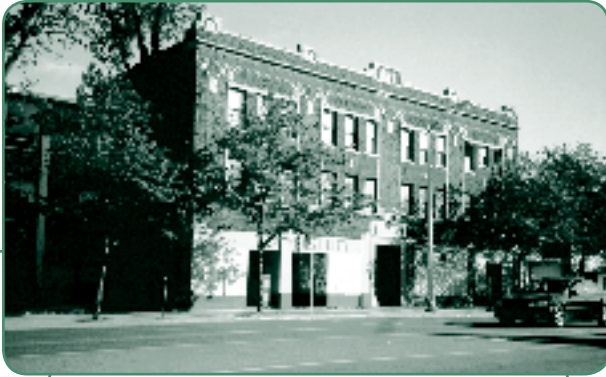
Vacant commercial building on East Jefferson slated for redevelopment
