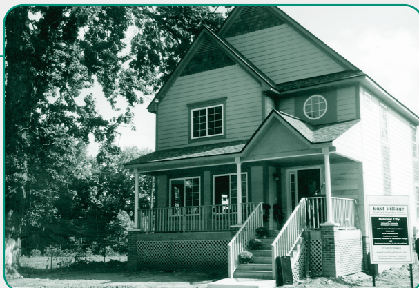
New construction in Detroit's East Village
